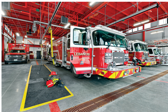
The interior vehicle bay was designed with LED lights and energy-saving ventilation systems. (Photo: Patrick Rogers)
