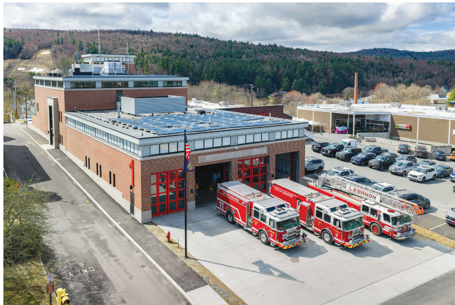
Lebanon, NH's Central Fire Station was designed to aim for net-zero-ready status which included solar, heat pumps, and RTUs on the roof. (ReArch)
